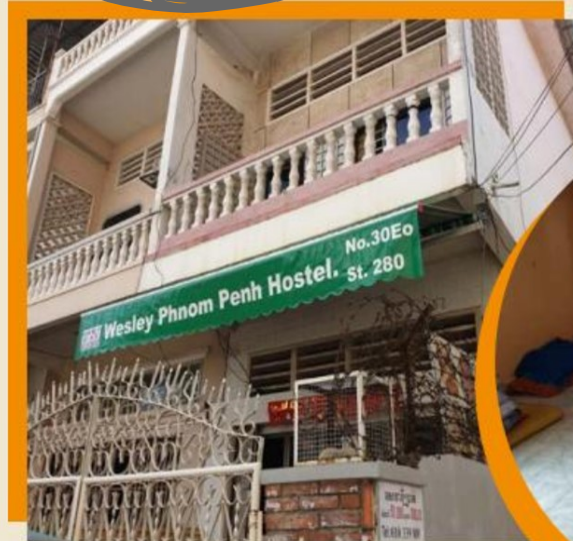
September 2019: Renovation completed
